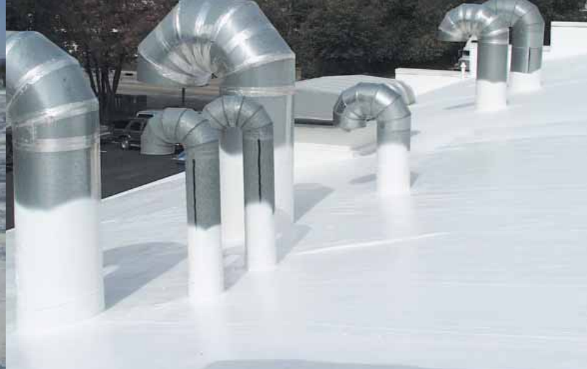
After: Completed restoration.
